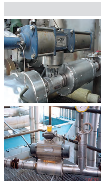
Pictured above are two thermal drains. These drain valves operate on temperature and can see a lot of cycles. ValvTechnologies has been successful in providing a solution for this application that provides repeatable, tight shut-off.
