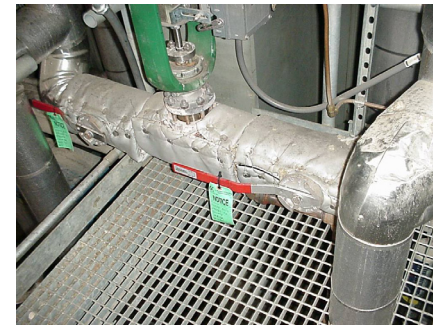
Installation of ValvTechnologies' high-pressure bi-directional valve
