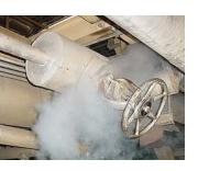
Globe type valves often develop dangerous leak paths due to their torque seated design. Their linear operation requires an operator to seat the plug by exterior force, often repetitively as the flow stream can cause the valve to become unseated.
